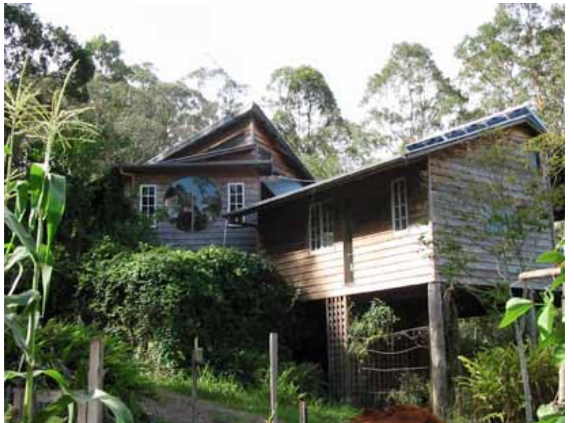
Fig 8. Solar House at Crystal Waters. Photo: Max O Lindegger
