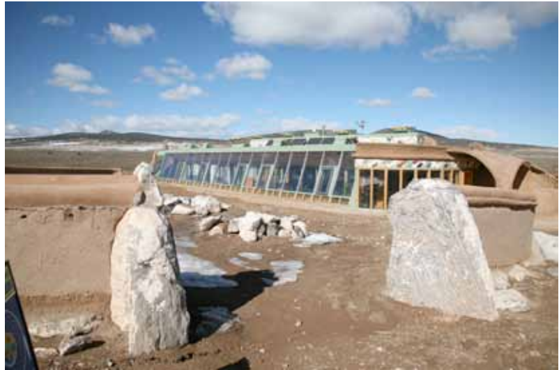
Fig 5. Corner Cottage Earthship at Taos, New Mexico. Photo: Kirsten Jacobsen
