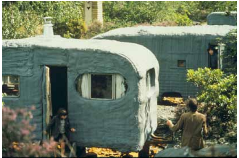
Fig 3. Caravans sprayed with insulation serving as site offices. Photo: Courtesy: CAT
