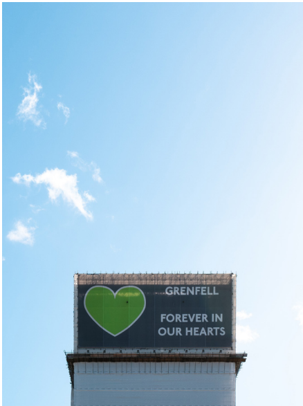
[Figure 1: Grenfell Tower]
