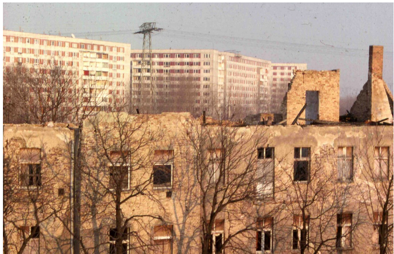
Fig. 3. 19th Century building fabric was neglected in East Berlin and replaced with apartment blocks (Plattenbau). Photo: Dougal Sheridan, 1994-1996.
