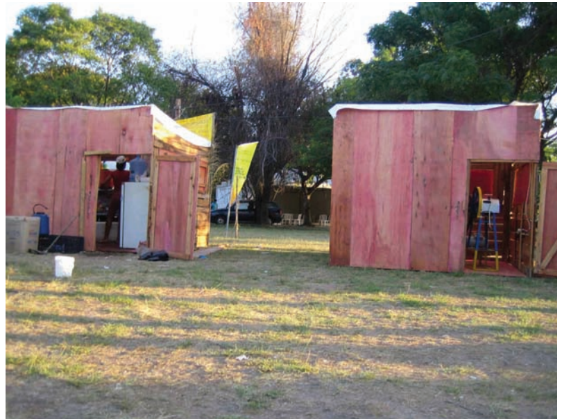
Fig. 3. Nova União Da Arte Workshop Space and its demolition in Vila Nova, São Miguel, Brazil. Photo: Mick O'Kelly, 2005.
