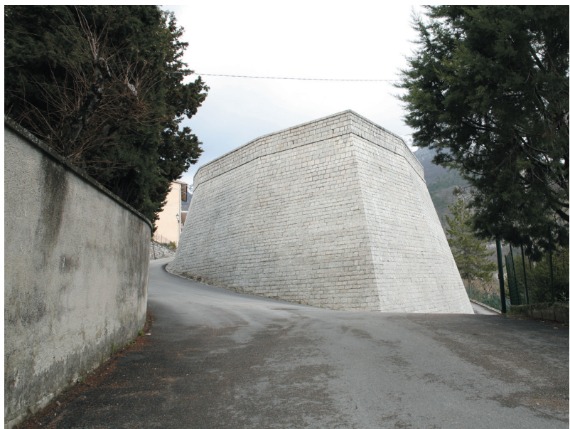
Fig. 1. Ravelin, Costacciaro, Umbria, Italy, by Francesco di Giorgio, 1477. Photograph: Tim Gough.
