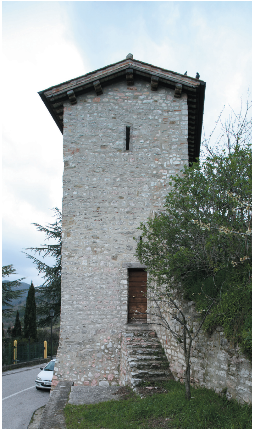
Fig. 2. Defensive tower, Costacciaro, Umbria, Italy, by Francesco di Giorgio, 1477. Photograph: Tim Gough.
