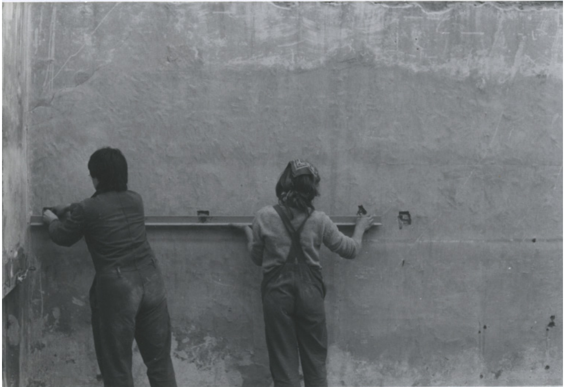
Fig. 6 Architects Mary-Lou Arscott and Susan Francis, one of the founder members of Matrix, setting out a floor plate. Photograph used with permission of Susan Francis
