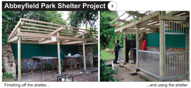
Fig. 5. Abbeyfield Park Shelter Project, nearly finished. Image: Bureau of Design Research.
