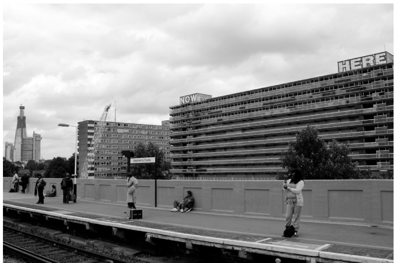
Fig. 4. Claydon block and intervention on its roof, Heygate estate, 21 September 2011. Author's own photograph.
